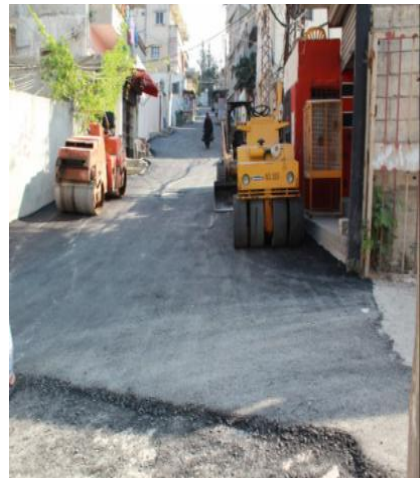
Water upgrading project in Beirut
