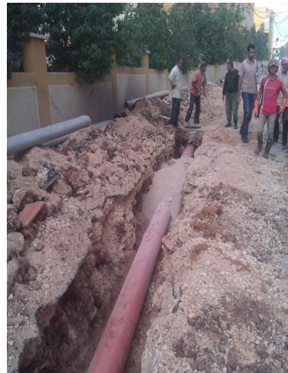
Sewage renewal project in Tyr
